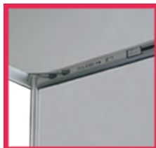
ISOLATOR WITHIN THE FITZIN CROSS
