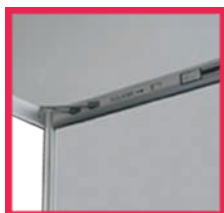
ISOLATOR WITHIN THE FITZIN CROSS
